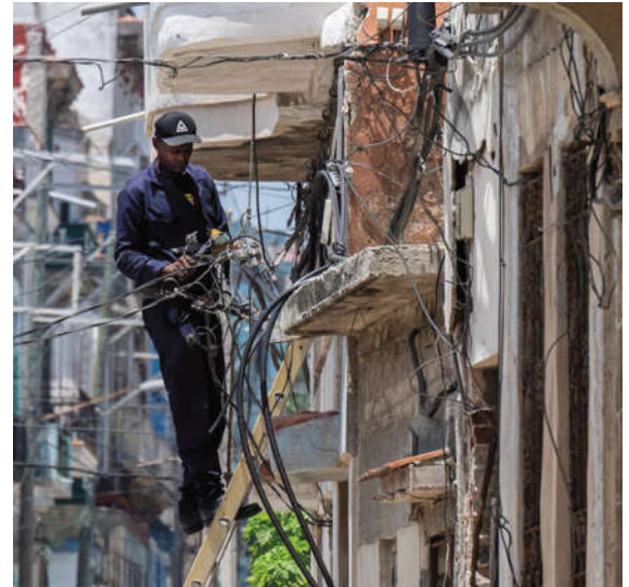
Cuban electrical workers repair power-generating equipment to restore electricity after a blackout. The U.S. blockade has left Cuba's power system short of fuel and replacement parts, but workers continue the struggle to keep the electricity flowing. Photo: Prensa Latina.
