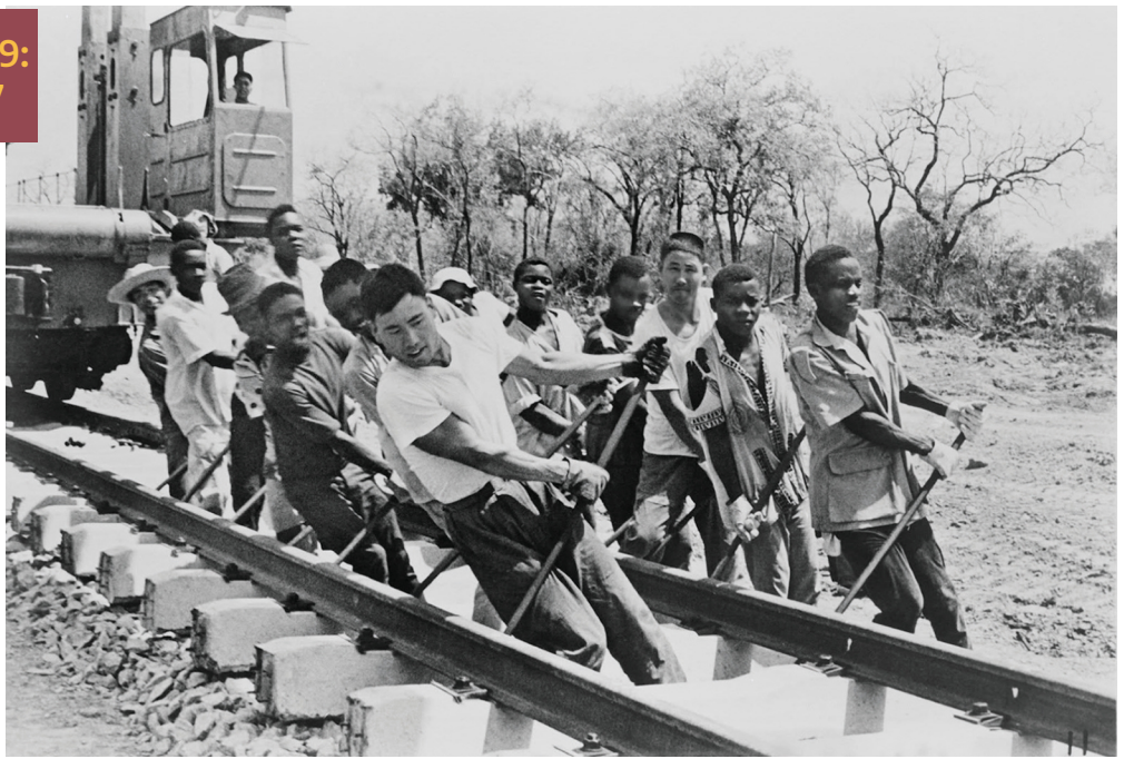
Chinese and African workers build the Tanzania-Zambia Railway in the 1970s. China helped construct the line so newly independent African countries could move goods without relying on routes controlled by apartheid South Africa and Rhodesia.
