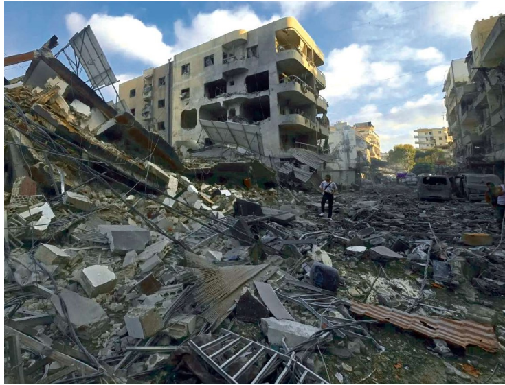
Site of an Israeli strike that hit near a hospital in the southern Lebanese city of Tyre on June 1, 2026.
