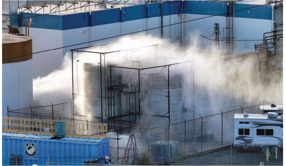
Water sprays over storage tanks at the GKN Aerospace facility in Garden Grove, California, after an overheating tank of methyl methacrylate forced 50,000 residents from their homes. GKN’s Garden Grove plant manufactures canopies for F-35 fighter jets and other military aircraft.
