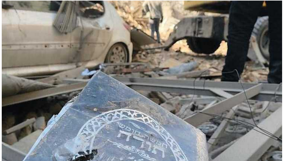
Photo of the damage to the Rafi Niya Synagogue.
