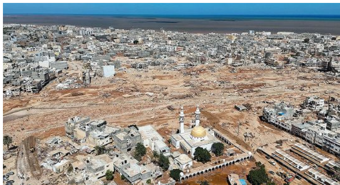
Floods devastated Derna, Libya.
