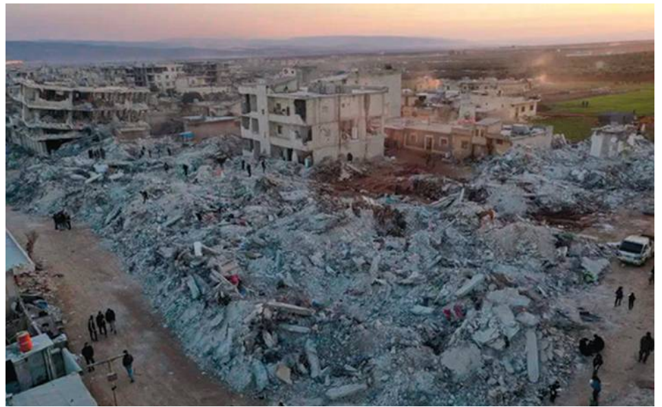
Collapsed buildings in the town of Jinderis, Aleppo province, Syria, Thursday, Feb. 9, 2023. The quake that razed thousands of buildings was one of the deadliest worldwide in more than a decade.
